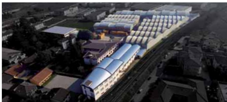
SCAB sede/headquarters - Coccaglio (BS) Italy
